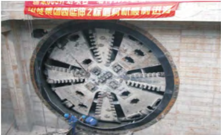
Shield Tunnel Boring Machine used on Shanghai subway
