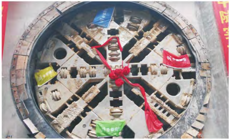
The cutting machine tool in Beijing metro line two,ten sand and gravel stratum
